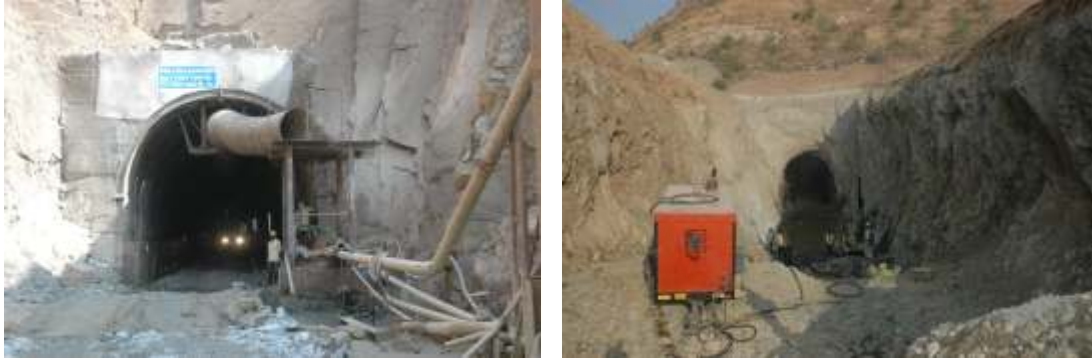
Stage II - Under Construction ( photographs as on 10.01.2009 )
