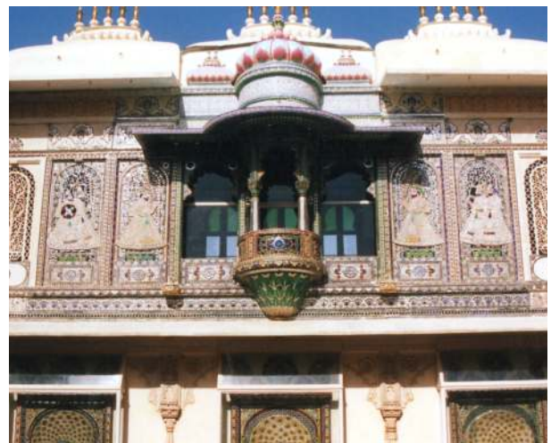
The Mor Chowk East Wall - Before
