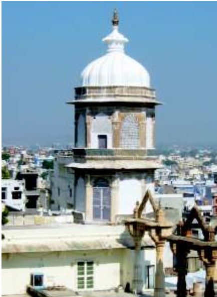
Nakkarkhana ki Chatri after restoration
