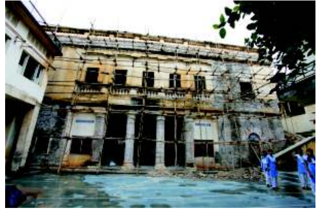
Restoration work in progress at the outer façade of the school building
