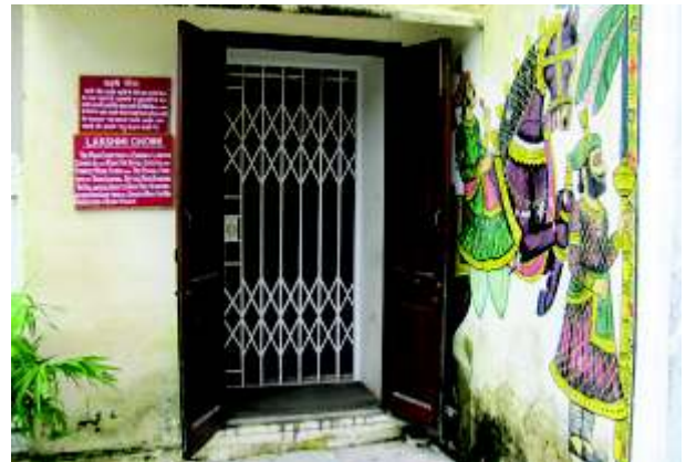
View of Lift at Laxmi Chowk
