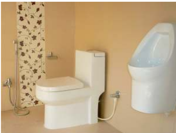
Bio-Digester Toilet System at Chota Darikhana, Ganesh Chowk, The City Palace Museum, Udaipur
