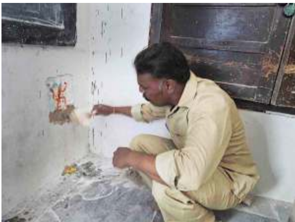
2nd phase of restoration and renovation in progress
