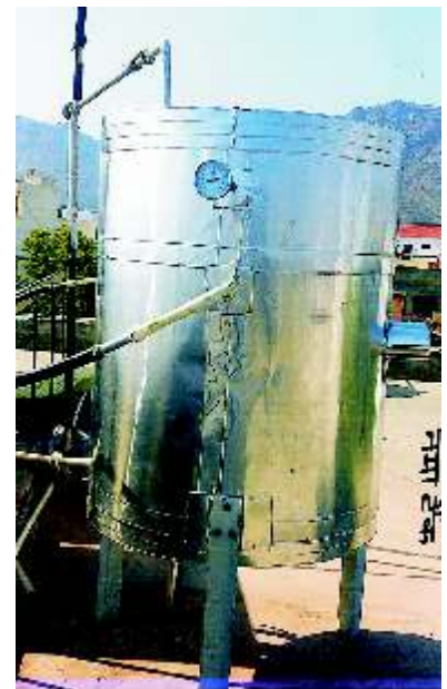
Newly installed Solar Water System at Badhir School, Vaishali Nagar, Ajmer
