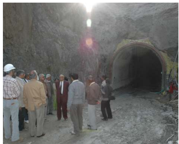
End Point of the Tunnel (Under Construction)
