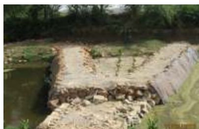
Bridge No. 4 with Ecofert
