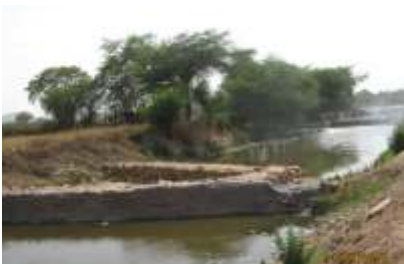
Bridge No. 2 back
