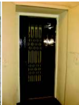
View of Lift at Sabha Shiromani ka Darikhana
