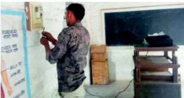
Technician fixing some IT fixtures at Ahilya Bal Jyoti School, Maheshwar, MP
