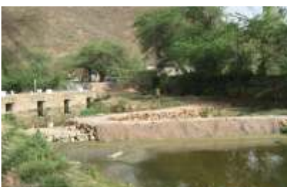
Bridge No. 4 front
